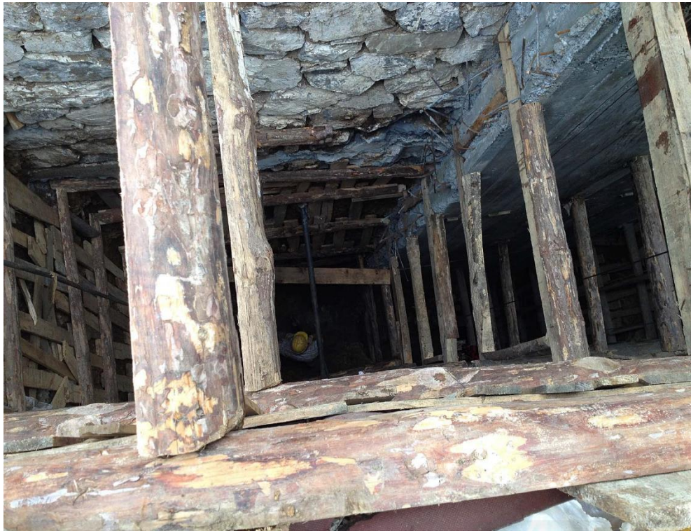
Figure 6: Partially completed wall and ongoing excavation at adjacent location
