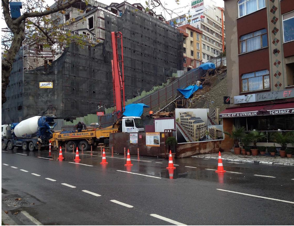
Figure 3: Early stage of construction at second lot
