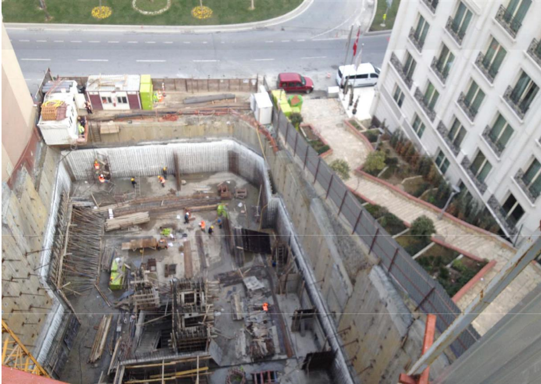
Figure 11: Ongoing main construction on second site
