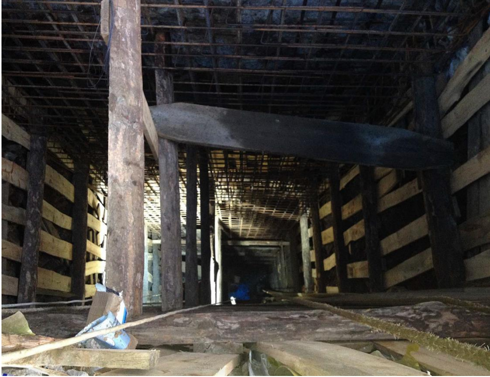
Figure 5: Reinforcement installation for the wall
